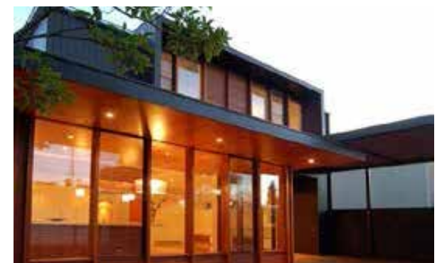
Fig. 10 - Passive design elements such as eaves/roof overhangs for temperature control
