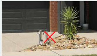
Fig. 76 - Positioned close to driveways
