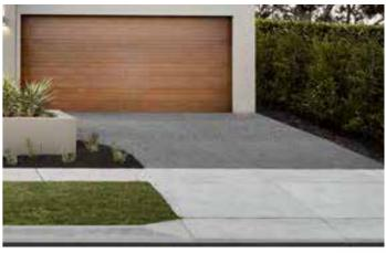
Fig. 28 - Internal driveway matches the crossover width
