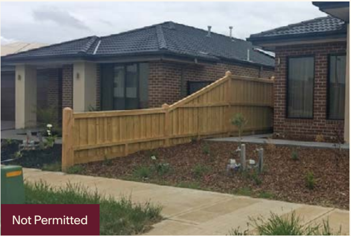
Fig 23 – Side fencing beyond dwelling is not permitted
