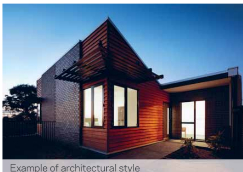
Example of architectural style
