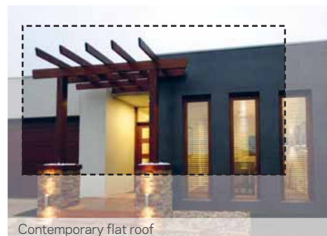
Contemporary flat roof
